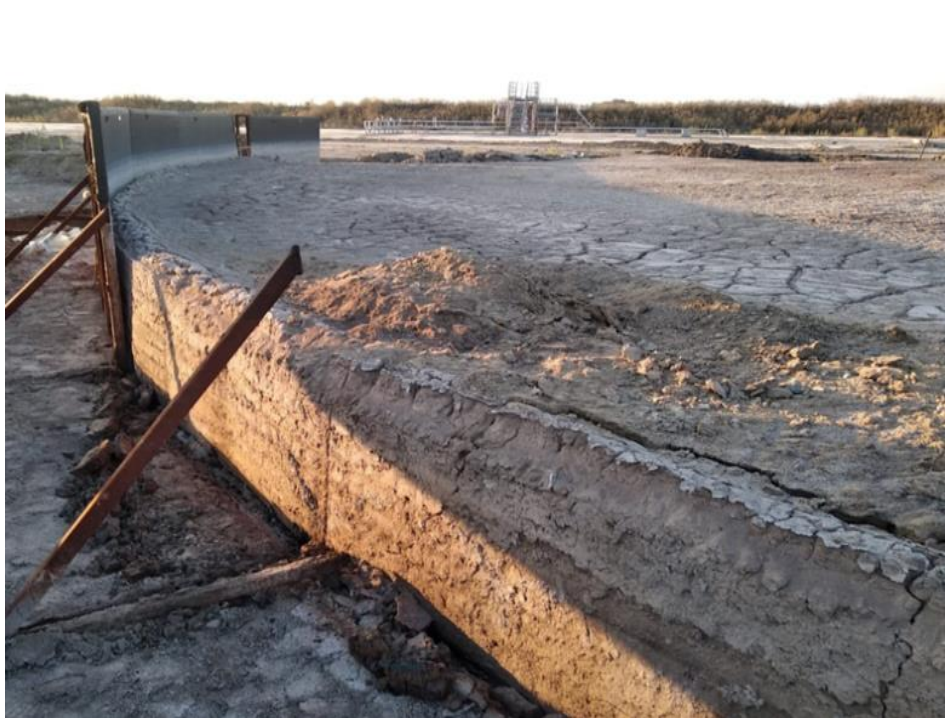
Fig. 3. Dry residue of drilling mud
