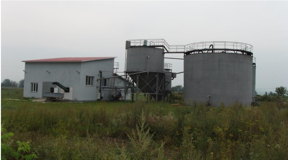
Fig. 4. Wastewater treatment plant of concentrate apple juice production plant in "Bukofruit"
