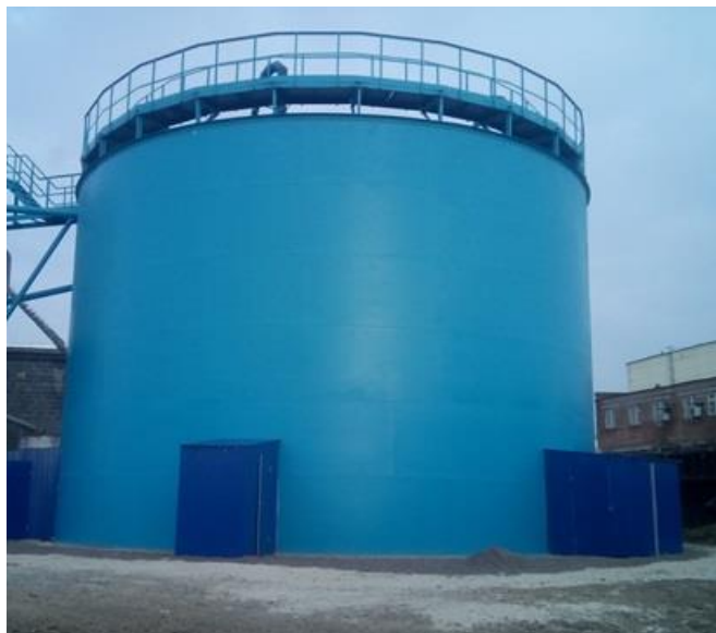
Fig. 11. Aerotank-settler with surface jet aeration
