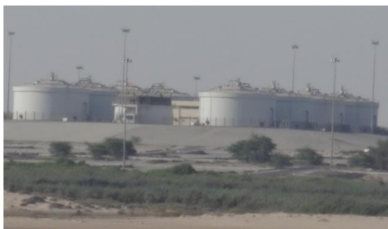
Photo 12. Mafrq sewage treatment plant. Closed sedimentation fermentation chambers (anaerobic digesters). UAE (photo by W. Sobczyk)
