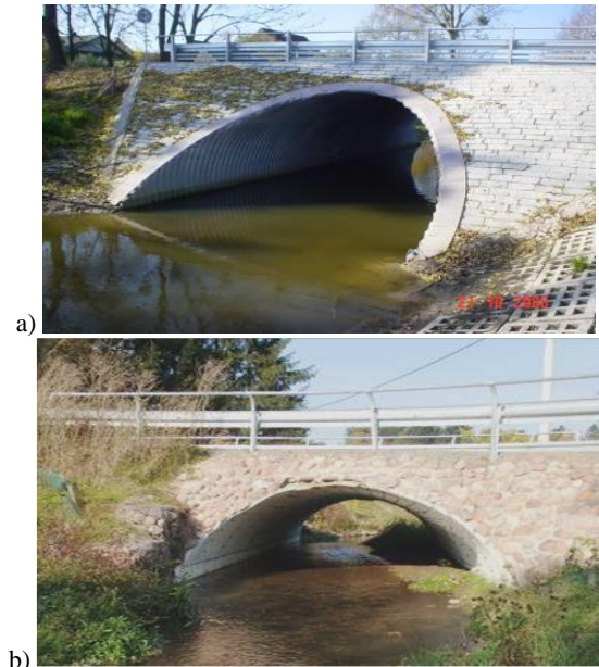
Figure 4. River culverts designed in accordance to old and new standards a) built in 2006 b) constructed in 2013
