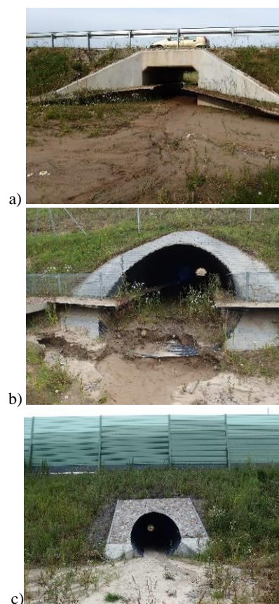
Figure 2. Culverts for small animals – shapes of clearance gauge a) rectangular b) parabolic c) circular
