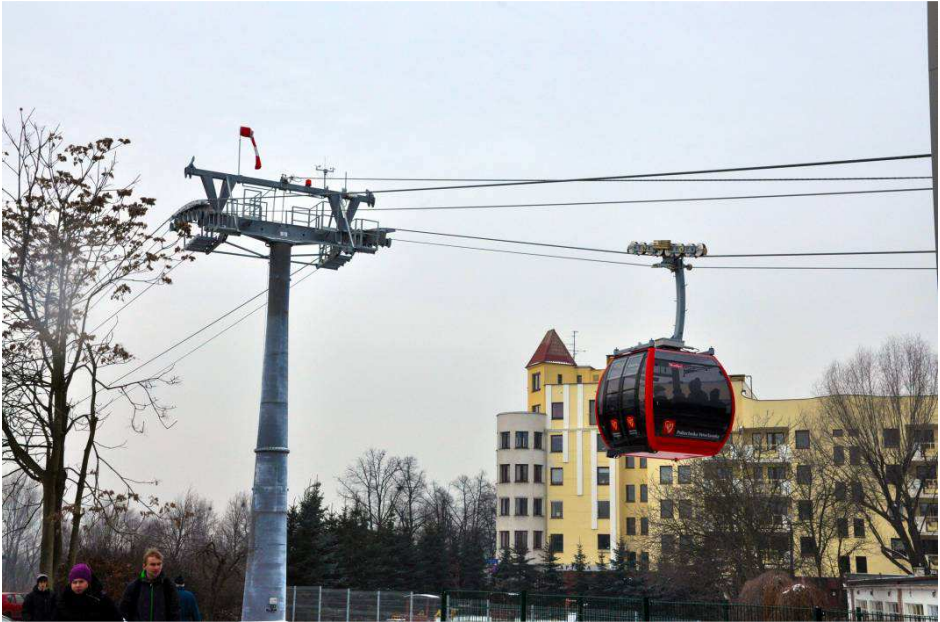
Fig. 148. Cable car 'Polinka' combining Main Campus and Geocentrum Educational-Research Unit Na Grobli street, phot E. Pol 2013.
