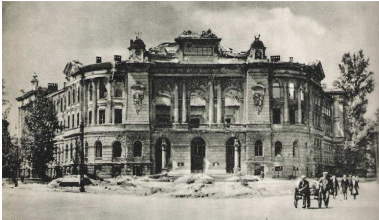
Fig. 11. Destroyed building of the Warsaw Technical University, 1945
