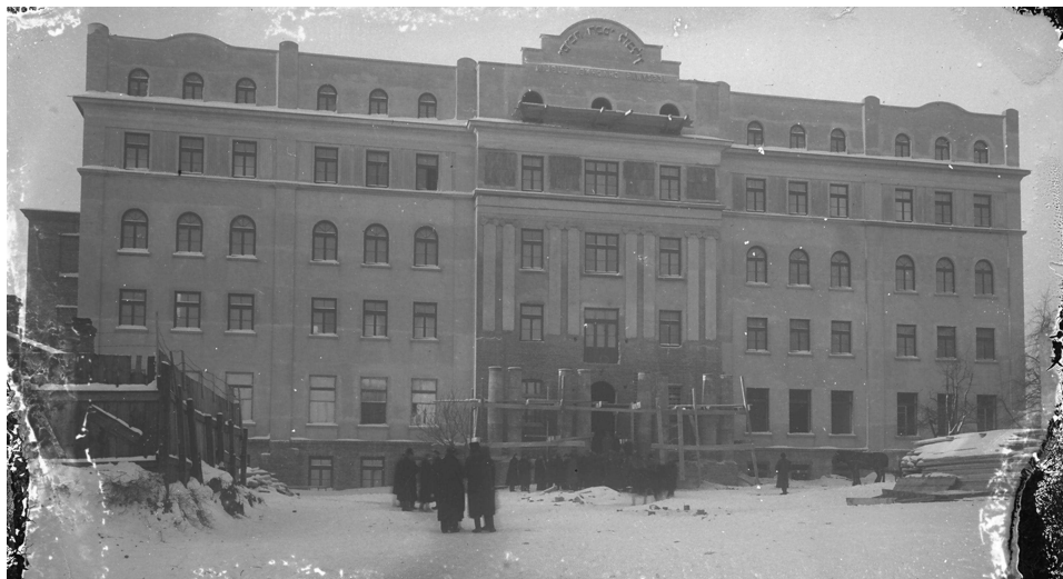
Fig. 105. Yeshiva building in 1927 during construction. Source: Photography Archive "Grodzka Gate - NN Theatre"
