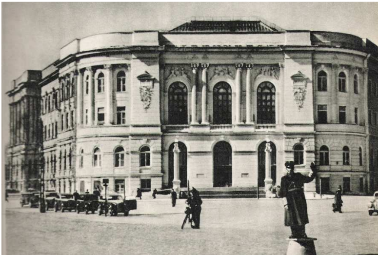
Fig.12. Building of the Warsaw Technical University, 1948
