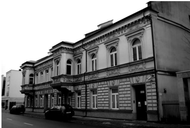
Fig. 92 Buildings at 1/3 3rd of May St. Warszawskiej50 - the seat of the Chair of Catholic Theology, University of Białystok. (photo by M. Kłopotowski)
