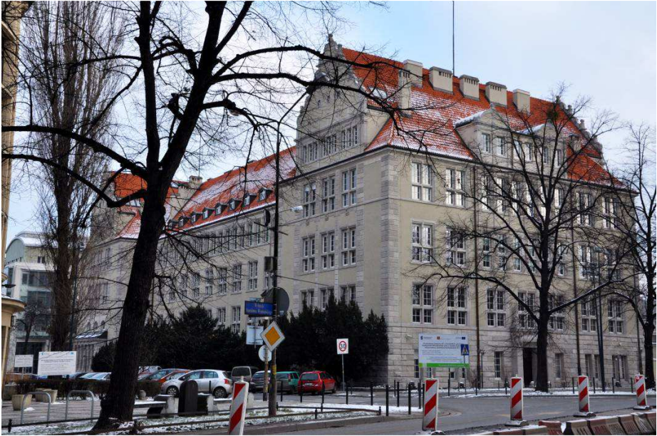
Fig. 140. B-1 building formerly belonging to the Institute of Metallurgy (E) from the S. Wyspiański shore, currently Institutes: Material Science and Applied Mechanics, Organization and Management, Inorganic Technology and Mineral Fertilizers, phot. E. Pol 2013.
