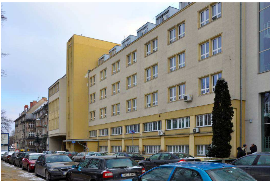
Fig. 143. Building B-5 built in the 1950s according to project of prof. arch. Andrzej Frydecki, phot. E. Pol 2013.
