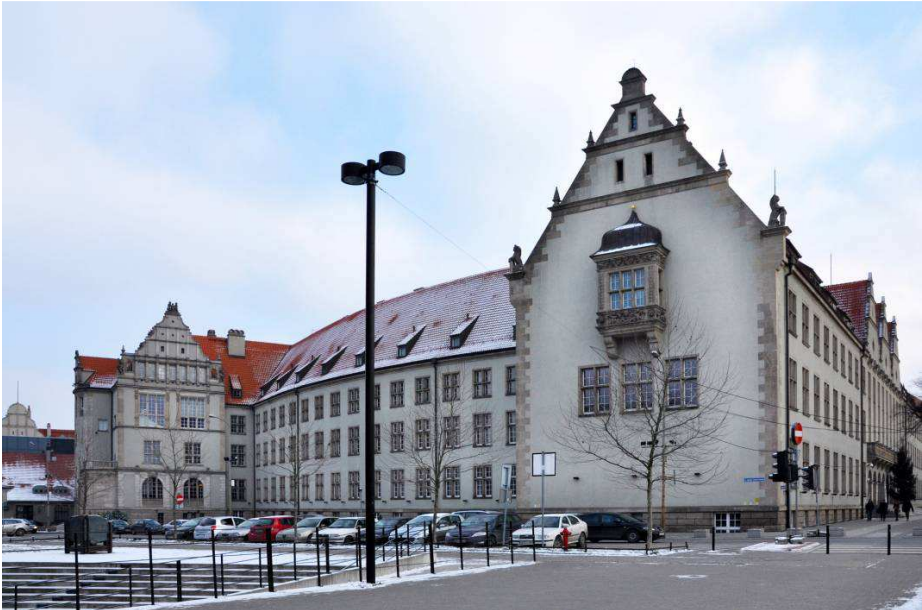
Fig. 142. Wing of the Main Building (A-1) from the C. K. Norwid street designed by Max Schimer and Heinrich Müller, phot. E. Pol 2013
