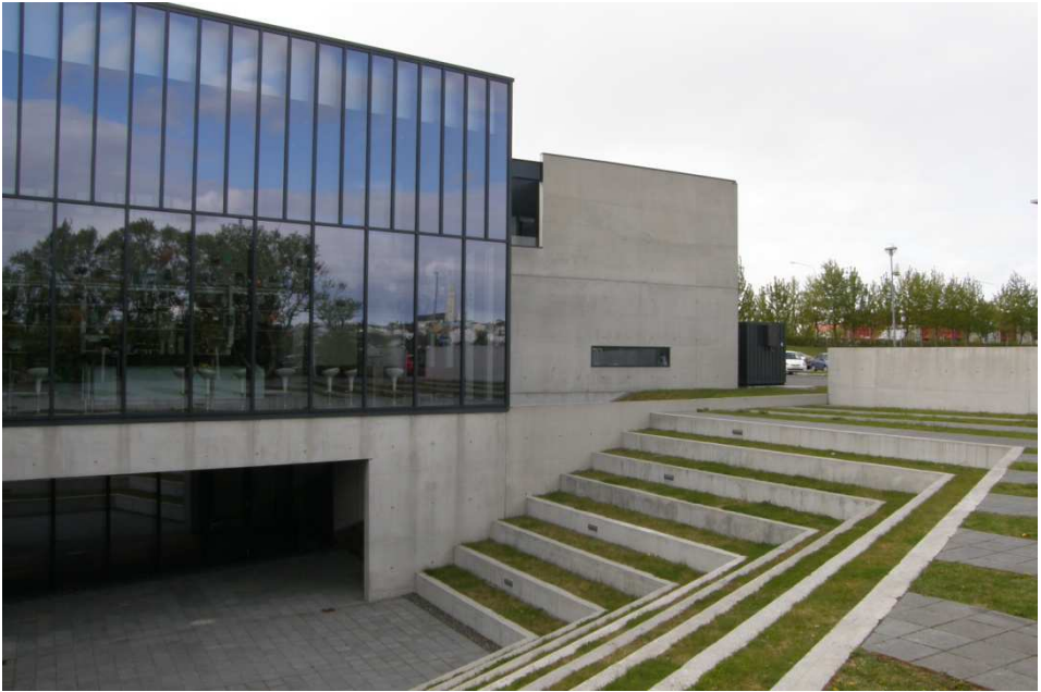
Fig. 4. Multi-purpose stairs in the campus of Reykjavik University. Photo by N. Przesmycka 2013.
