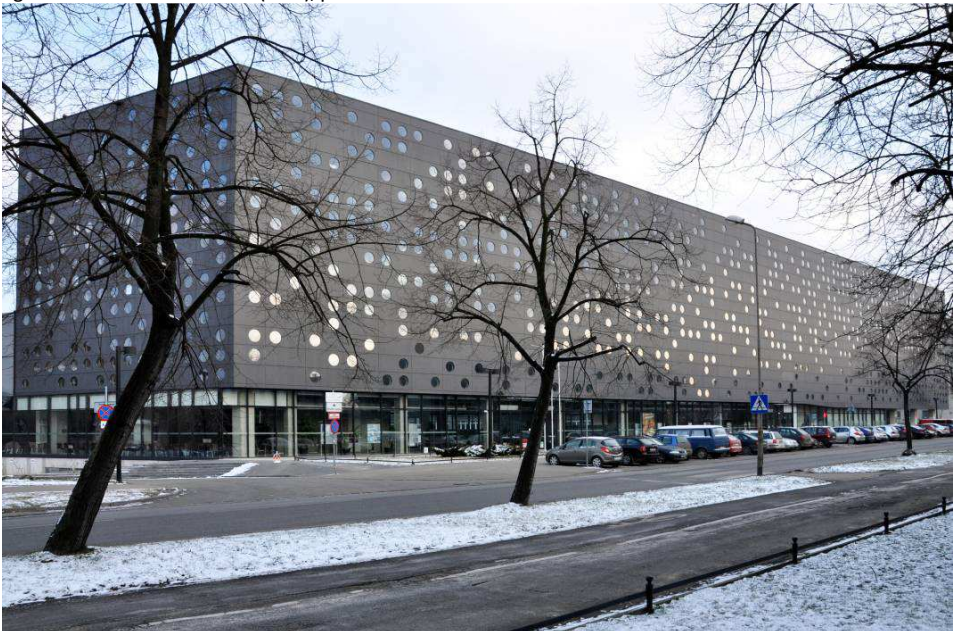
Fig. 150. Building of Students' Integrated Center (C-13), phot E. Pol 2013.
