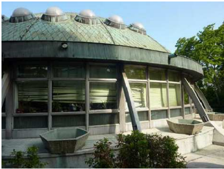
Fig. 118. The ophthalmology auditorium before modernization works
