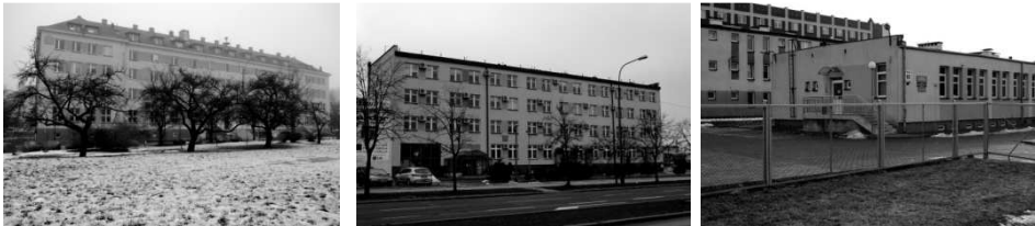
Fig. 91. Buildings Department of Biology - Chemistry UwB: ul. 20B Świerkowa Street, 1 Hurtowa, 65 Pogodna Street (photo by M. Kłopotowski)
