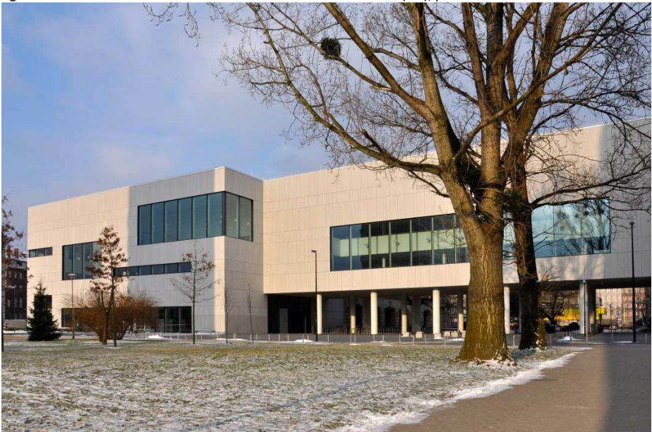
Fig. 152. Building of Library of Science and Technology 'BIBLIOTECH' (D-21), phot E. Pol 2013.
