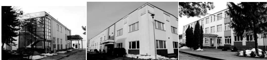
Fig. 55, 56, 57 Dean's Office, Buildings Teaching Berlin and Philadelphia belonging to the Faculty of Management PB. (photo by M. Kłopotowski)
