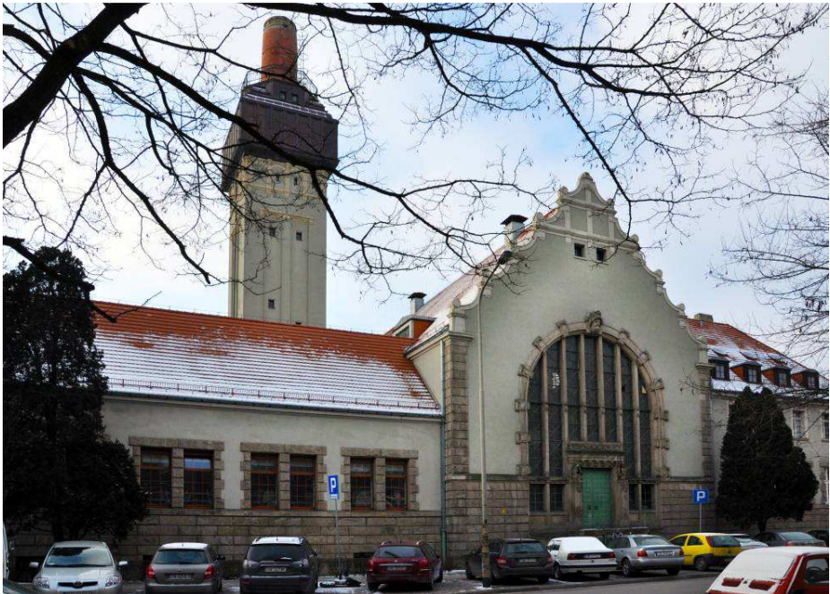
Fig. 138. A-4 building of former dawniej Machine Laboratory (C), now the Institute of Heat Engineering and Fluid Mechanics, phot. E. Pol 2013.
