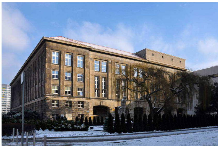
Fig. 145. Building D-2, phot. E. Pol 2013.
