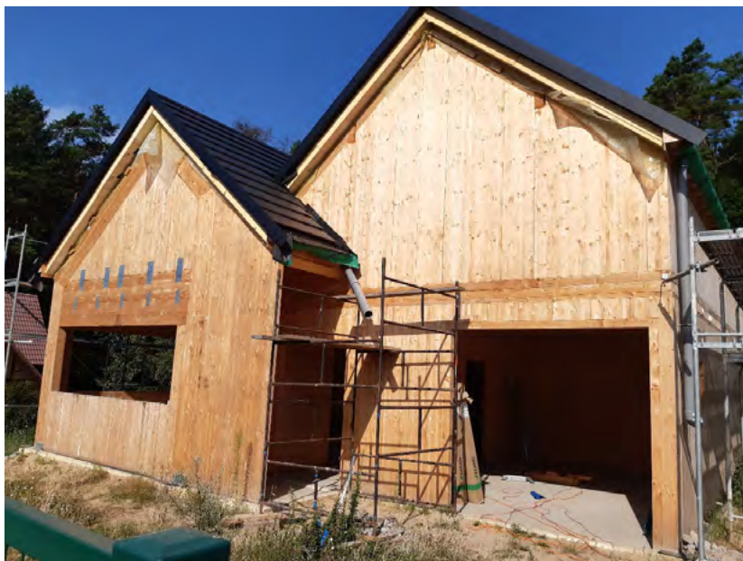
Fig. 2. Building in a wooden structure. Own photo
