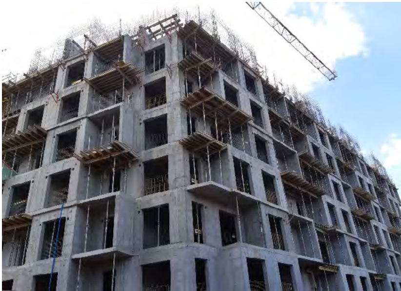
Fig. 1. Reinforced concrete structure. Own photo
