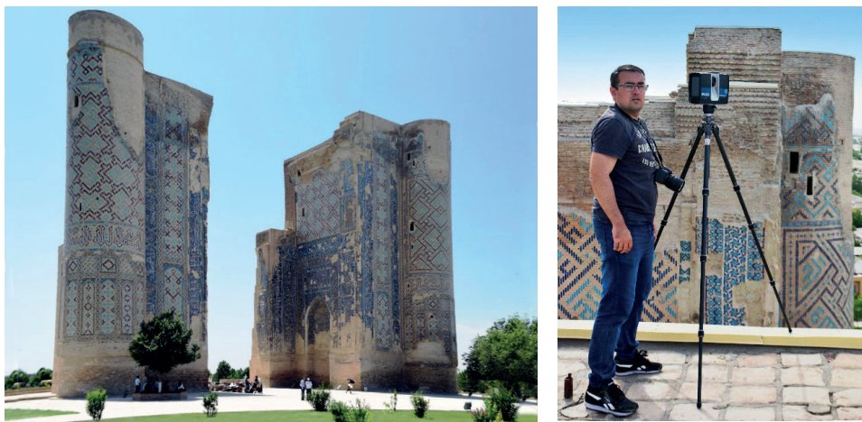
Fig. 26. View of the remains of the ajwan of Timur's palace and its 3D scan in 2022. By the authors
