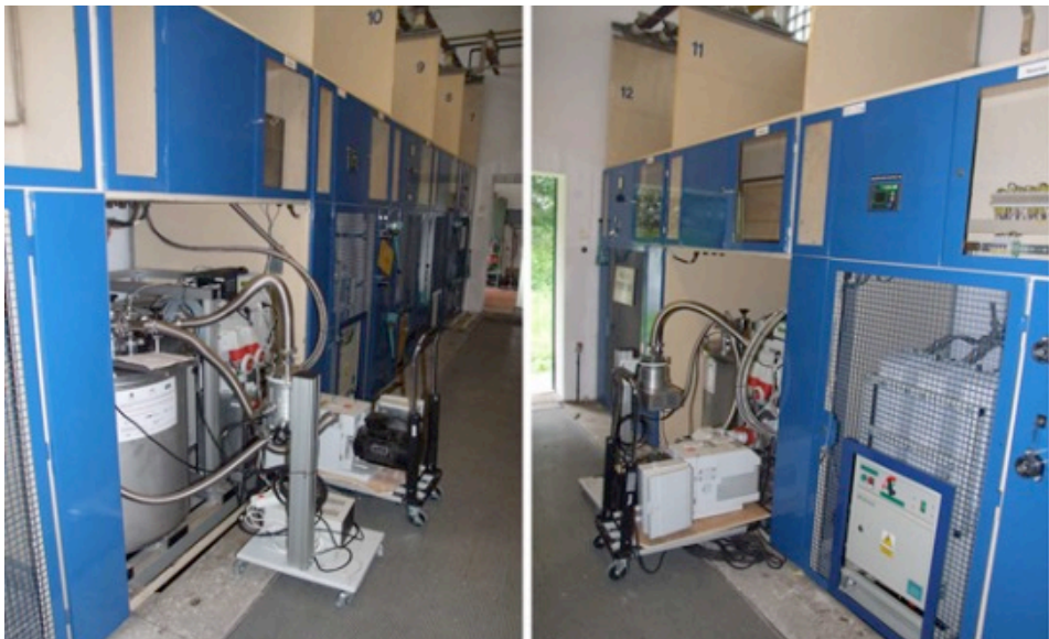
Figure 6.20. A superconducting current limiter installed in GS2 110 kV/6 kV switchgear on the premises of the Electrotechnical Institute. Source: own elaboration
