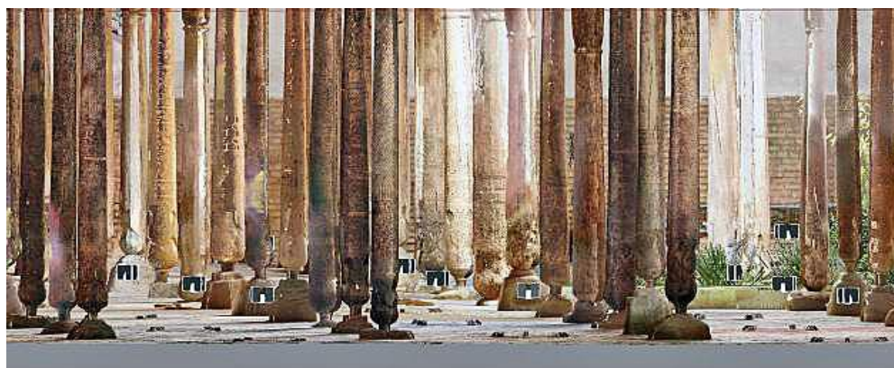
Fig. 5.11. The shape of the columns in the Juma Mosque – point cloud after multiple partial scans. By the authors
