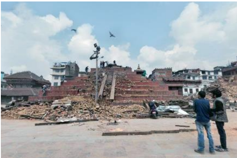
Fig. 1.10. Temple at Patan Durbar Square: (a) before, (b) after the earthquake [10]
