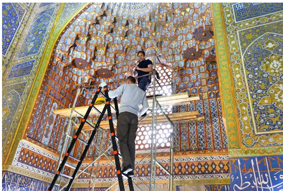
Fig. 4.5. Stalactite scanning at the 7 m height above the floor, 2019, Sher-Dor Madrasah, Registan Ensemble, Samarkand, Uzbekistan [4]
