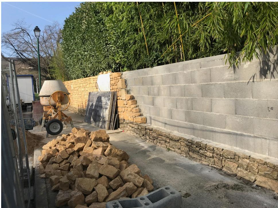
Fig. 7 : Construction of a concrete wall with a stone facing near the site, © Author, 19.2.2021
