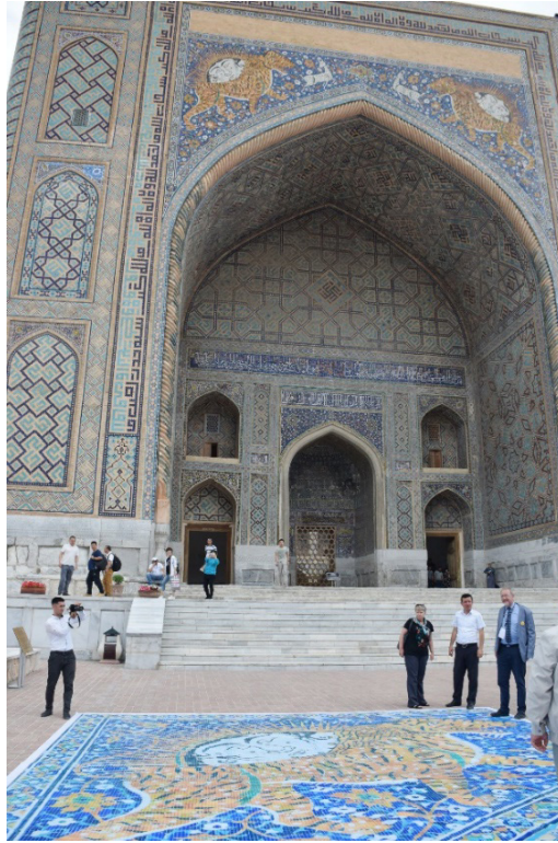
Figure 1. Fragment of a printed matrix in 1:1 scale for renovation of the mosaic in the Sher-dor Madrasa, prepared by staff of the Lublin University of Technology, photo: J. Montusiewicz
