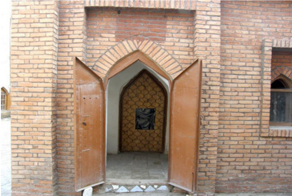
Figure 2. Entrance door to the Anushakhan bathroom [own source]
