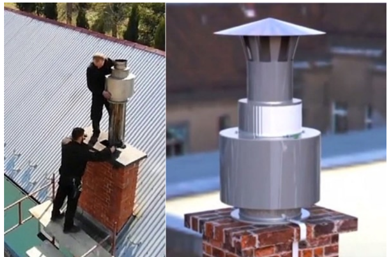
Fig. 3. View of the electrostatic precipitator prototype for home use
