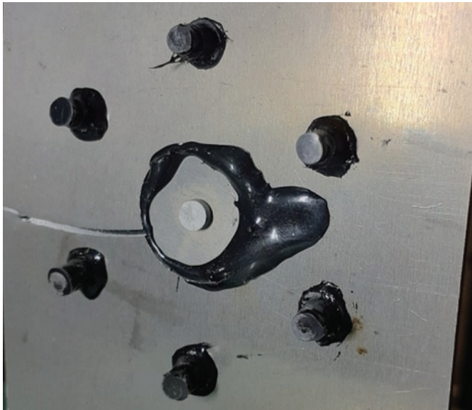
Fig. 25. Fatigue damage of a hybrid strapped joint (MBF2110AB-05-150 rivets and Raychem S1125 compound with a layer of Synglass E81 fabric)
