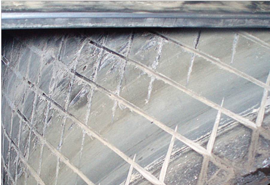
Fig. 17. Condition of the drive drum lining during the tests
