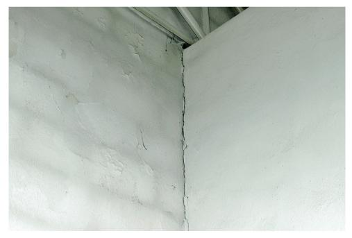
Fig. 11. Cracks at the junction of the masonry partition wall of the second storey with the western gable wall. Source: author
