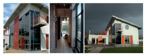
Fig. 2. Single-family building in Bytom: solar facade as an element of a passive solar system. Source: author
