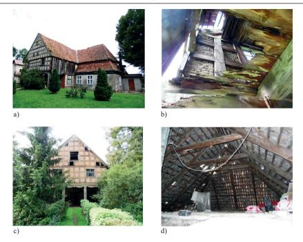
Fig. 6. Houses in: a) Steblewo 22/24, b) Steblewo 22/24 the catastrophic condition of the gable wall of the portico, c) Steblewo 15/17, d) Steblewo 15/17 leaking roofing (*photo by the author*)
