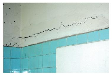
Fig. 10. Horizontal cracks in masonry partitions in basements. Source: author
