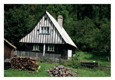
Fig. 2. The village of Młoty in the Bystrzyckie Mountains. A rural residential building with log walls, a gabled roof covered with sheet metal, with a slope of 45 degrees. *Photo by Jacek Suchodolski 2005*
