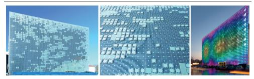
Fig. 4. Xicui Entertainment Hall in Beijing: solar facade as a screen composed of PV modules and LED lighting. *Source: Simone Giostra*
