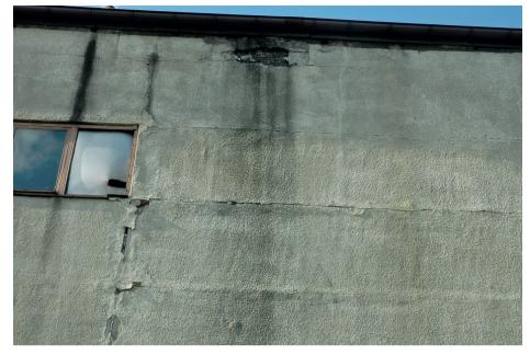
Fig. 12. Western fragment of the northern wall of segment 1 – visible cracks and chipping cracks and chipping of plaster at the joints of prefabricated housing elements and dark damp patches. *Source: author*
