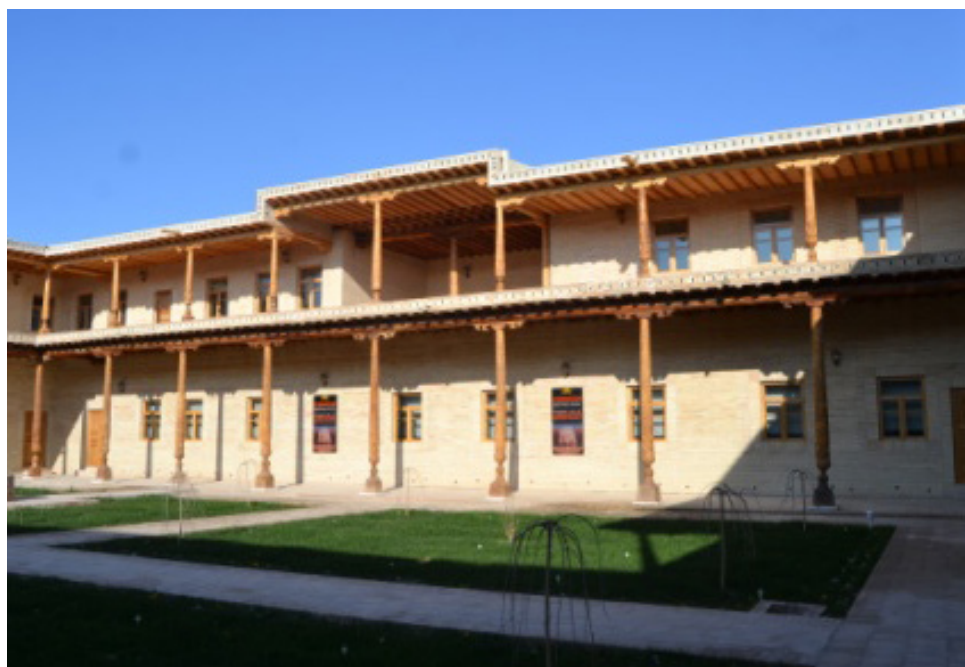
Fig. 3. 3 rd yard of Nurullabay complex. Current status. By the author (2021)
