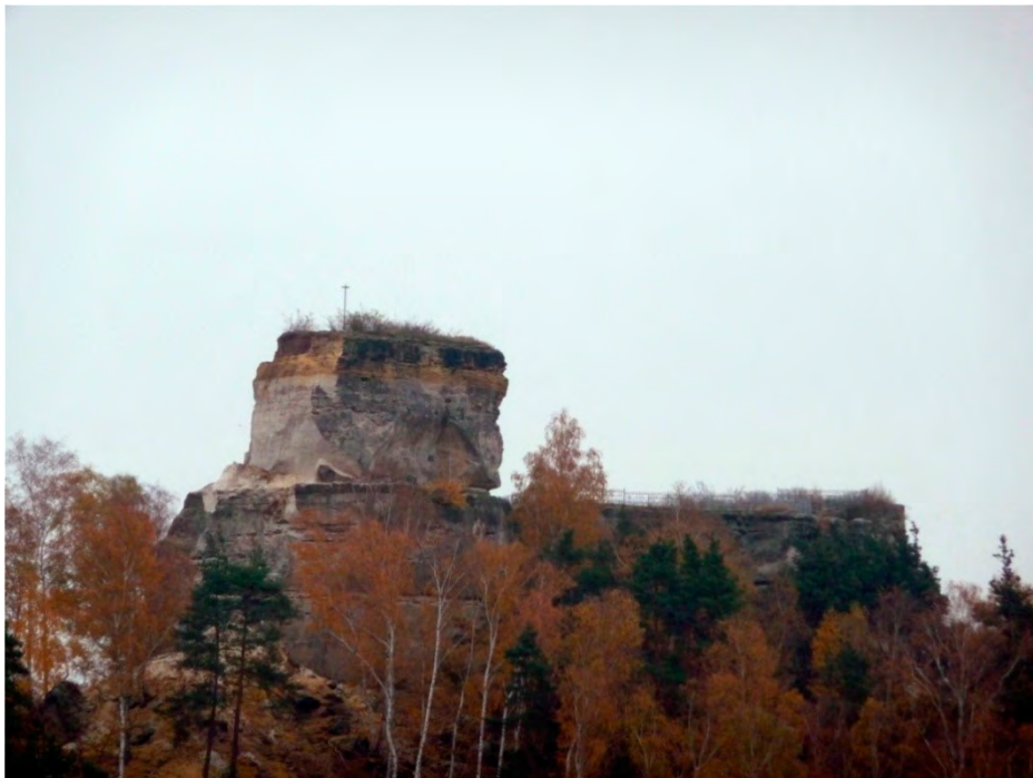
Fig. 38. Jestrebi Castle after the collapse, 2009.
