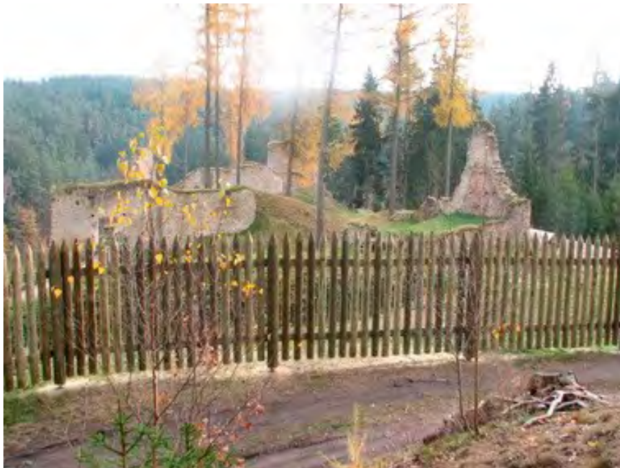
Fig. 20. Pořešín Castle, cleaned and stabilised, 2012
