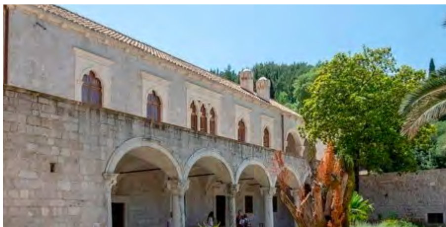
Fig. 10. Renovated villa of Bunić Kaboga family, Dubrovnik.
