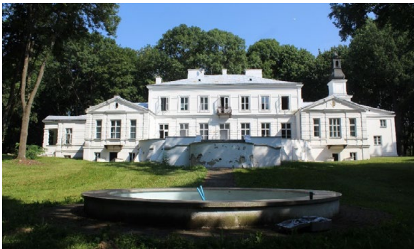
Fig. 2. South façade. (author's own photograph)
