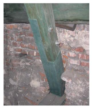
Fig. 2. Replacement of the rafter support zone with a new wooden part (photo. A. Halicka)
