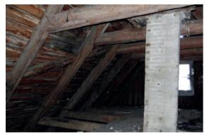
Fig. 10. Marynowy – the view on the rafter framing with two collar beams (author's own photography)
