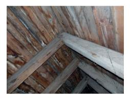
Fig. 13. Nowa Kościelnica - connection of the rafter (author's own photography)
