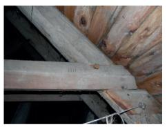
Fig. 14. Nowa Kościelnica - connection of the rafter with the collar beam(author's own photo.)
