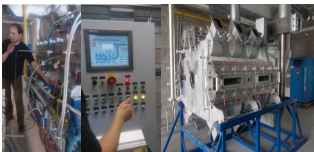
Fig. 2. Exterior installation digester
