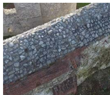
Fig. 5. Photo 3 Shaping the crown of the wall
