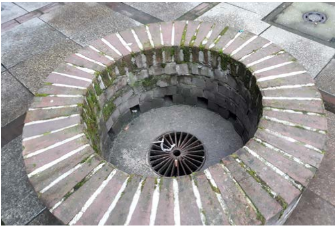
Fig. 8. Courtyard No. III, sewerage inlet built over by a brick circular piece of small architecture; Source: author's own photo
