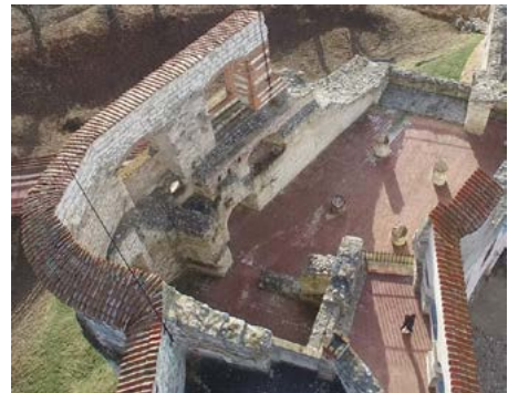
Fig. 7. Photo 4 Shaping the crown of the wall
