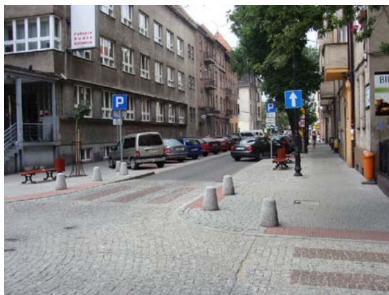
Fig. 5. & 6. Intersection of Juliusza Ligonía St. and Królowej Jadwigi St. in the centre of Katowice. The surface of the intersection is elevated to the level of the pavement and marked by paving. Source: photo by Hubert Trammer, August 3 rd , 2014.
