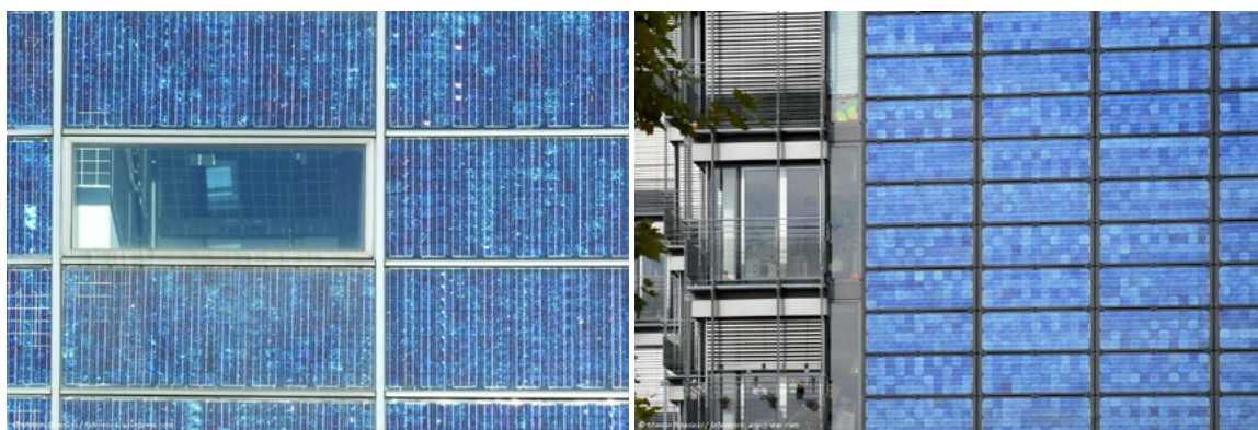
Fig. 2. Possible use of different types of cells on facades: a) monocrystalline (m-Si) cell used in the building in Punkthäuser Wilmersdorfer Straße, Freiburg (arch. Rolf + Hotz architekten, 2001, b) polycrystalline (p-Si) used in the building in SMA building nr 6, Niestetal (arch. HHS Planer+Architekten AG, 2002) – photographs by M. Muszyńska-Łanowy.
