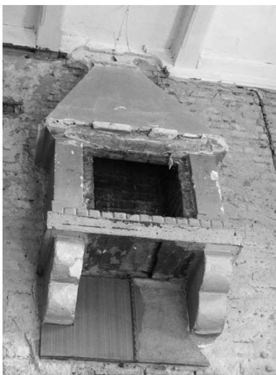
Fig. 7. Tatarów. "Straszny Dwór" guesthouse. Southern avant-corps , fireplace in the level of the first floor. Photo J. Czubiński, 2012.
