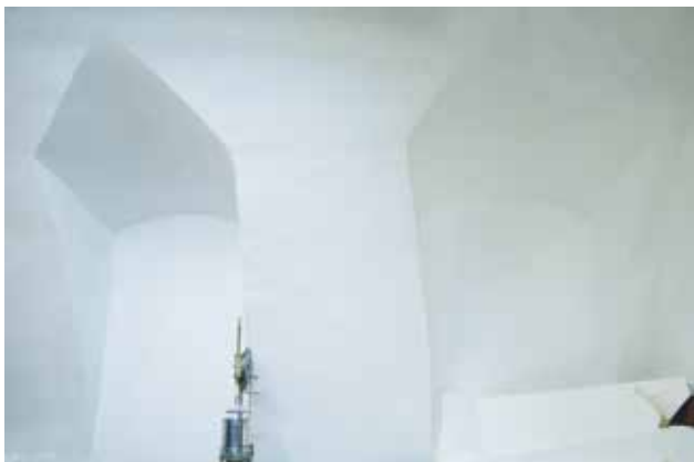
Photo 50. Paper mill building – barrel vault with lunettes in the lower ground floor. Photo by A. Fortuna-Marek
