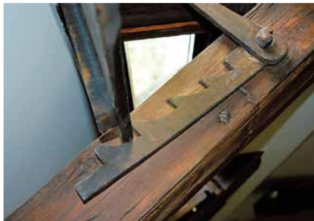
Photo 54. Flaps for regulating air flow Photo by A. Fortuna-Marek
