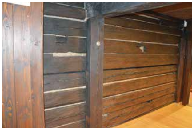
Photo 53. Log cabin structure of the oldest part of the drying house. Photo by A. Fortuna-Marek
