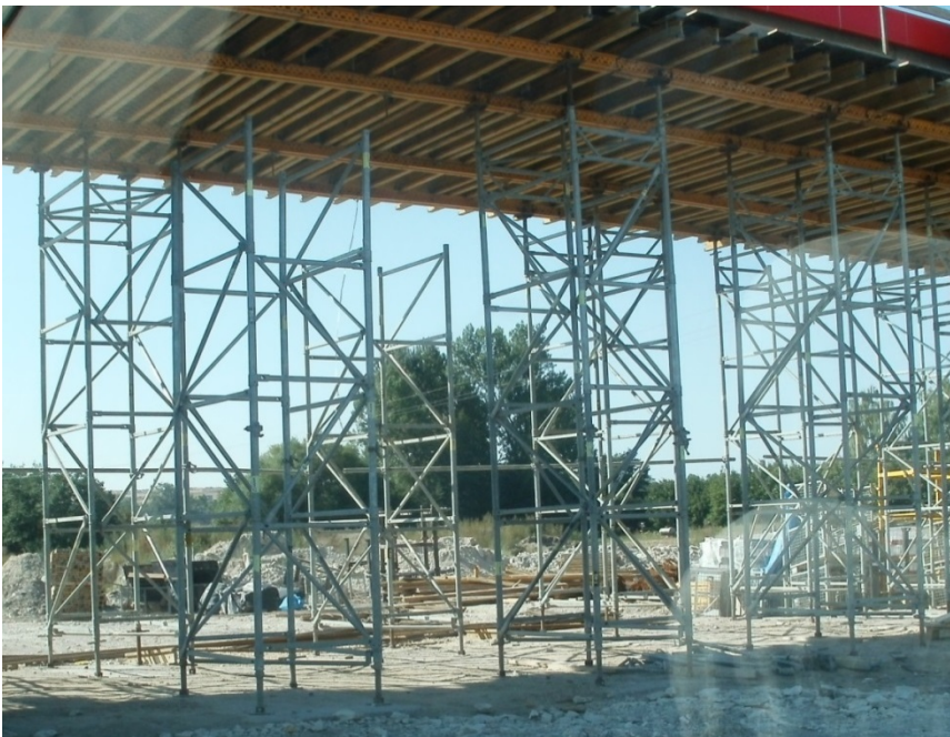
Fig. 2.11 The example of tower scaffold
