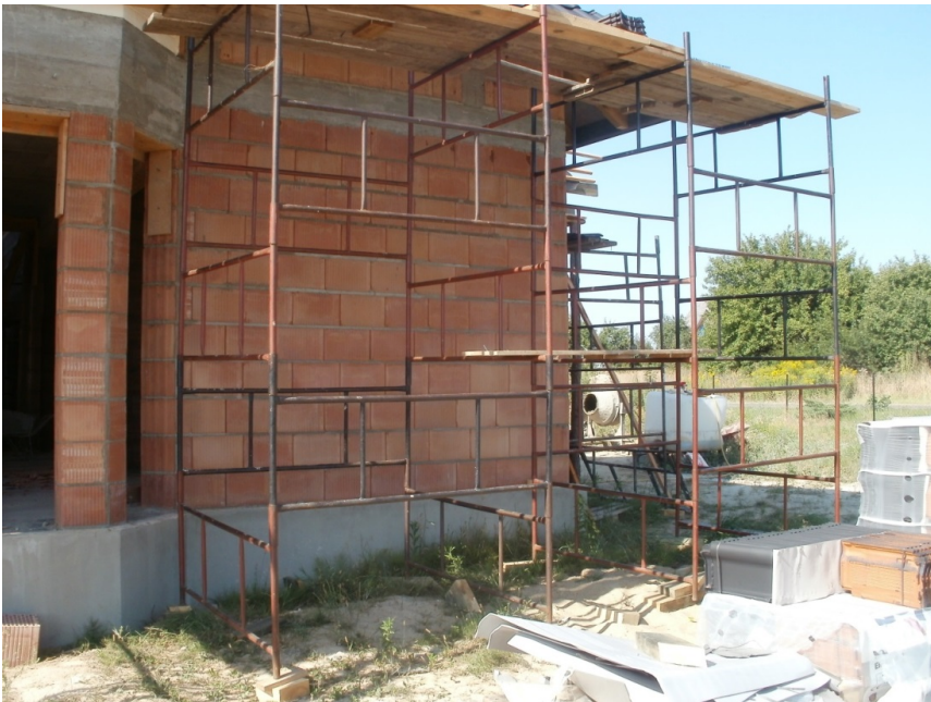
Fig. 2.7 The example of “warszawskie” scaffold
