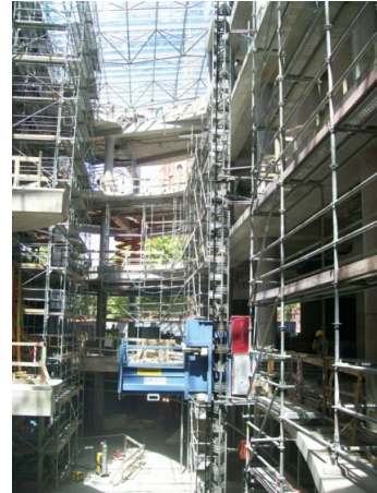
Fig. 5.2 A scaffold in the AGORA Shopping in Bytom Centre: a) static scheme; b) a scaffold during assembly conducted by Altrad Mostostal – Montaż
