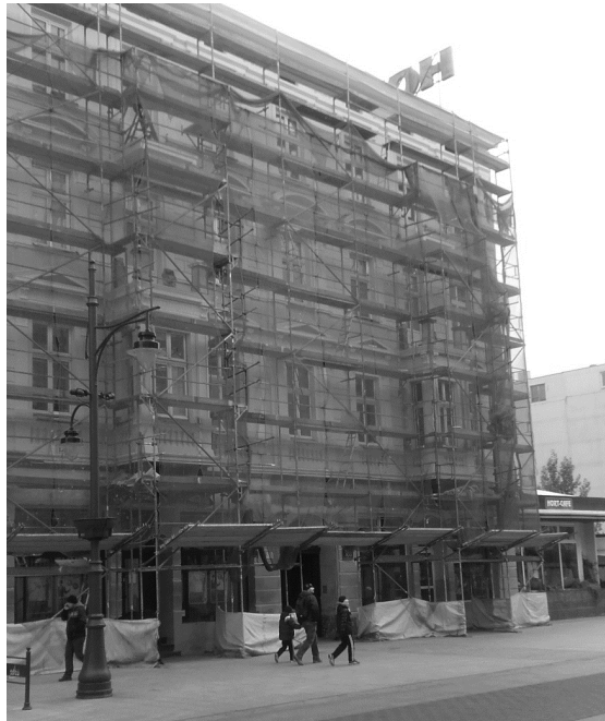
Fig. 2.12 The scaffolds with a safety net and protective fans
