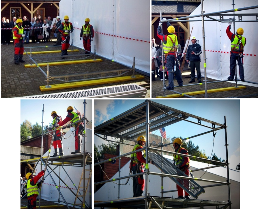
Fig. 3.11 The scaffold assembly
