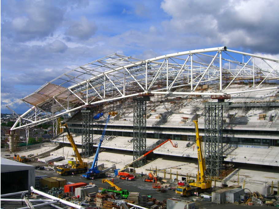
Fig. 2.11. Horseshoe truss construction process [www.grasshopper3d.com]
