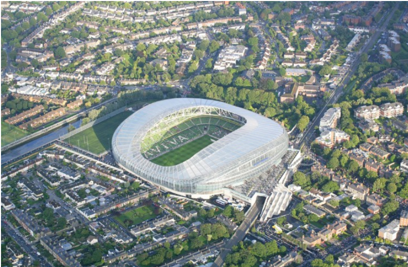
Fig. 1.3. Aviva Stadium in Dublin, Ireland [ www.avivastadium.ie ]
