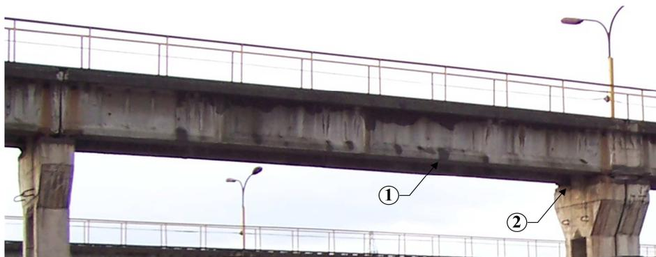
**Fig. 5.6.** View of precast RC crane beam; 1 – precast crane beam, 2 – two-branch column (photo by author)
