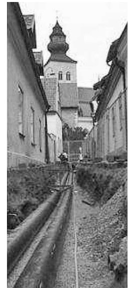
Fig. 5 District heating installed below the streets of the city centre of Visby, a World Heritage Site
