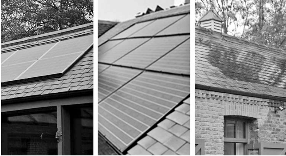
Fig. 4 Three photovoltaic panel systems with different heritage significance impact: The left photograph shows raised panels mounted on top of the roof covering, the mid-photo is of in-line panels and the right has solar slates.
