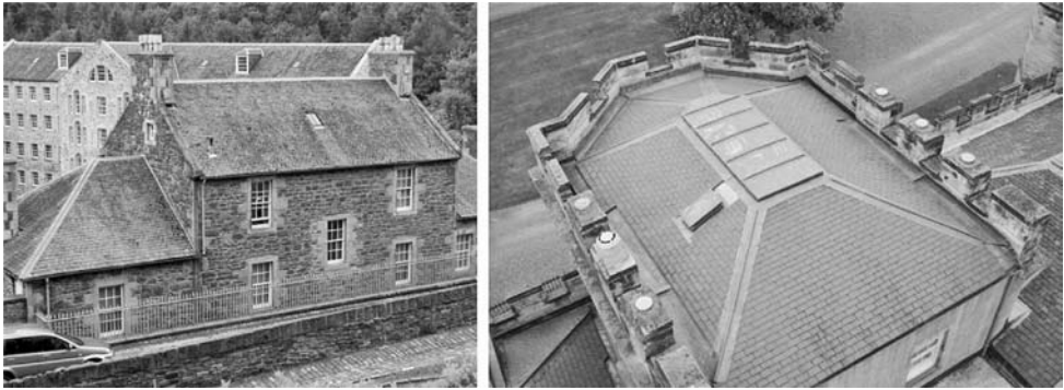
Fig. 3 The roof in the foreground of the left photograph has its original 18th century slates, visible from common viewpoints, whereas the roof covering on the right photo is a replacement, hidden behind a parapet.
