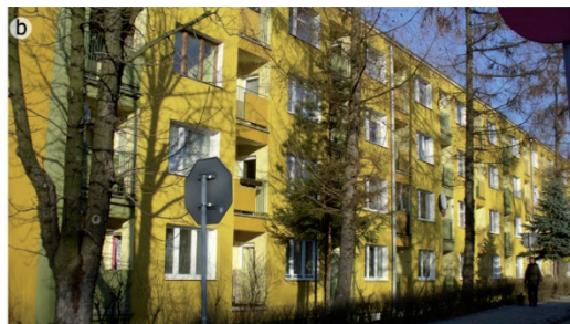
Fig. 9. Photos of a) north and b) south elevation, June 2011
