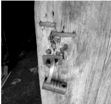
(Pic. 7) State of security elements – direct threat of burglary (photography depicting a wooden property inscribed on UNESCO's World Heritage List – yet, does not concern the churches in Lesser Poland Region), author: A. Fortuna-Marek
