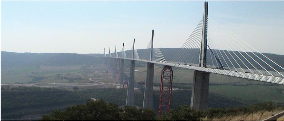
Figure 4.8.5. Overpass Millau, is a cable-stayed bridge that spans the valley of the River Tarn near Millau in southern France (by ALT).
