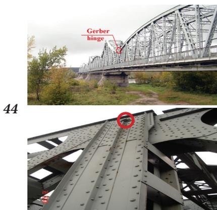
**Gerber scheme.** In the city of Puławy the old steel road bridge was built according to Gerber scheme in 1934. The shape of the upper truss belt corresponds to the graph of bending moments caused by permanent loads. The truss is not a continuous one. This is the so-called Gerber scheme. The Gerber hinge is circled in the illustration.
