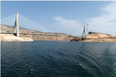
**...under construction.** The Nissibi Euphrates Bridge under construction. The side cables are fixed to the ground through the concrete deck. The main span is made of steel segments mounted sequentially as short cantilevers. Both pylons are made of concrete.
