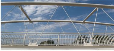
**Arch bridge.** A steel arch bridge with Nielsen (inclined) hangers. The foot-bridge in Szczeczeszyn.
