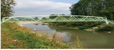
**Warren truss bridge.** The diagonal truss system (cross braces) resembles the letter W, often supplemented with hangers and posts.
