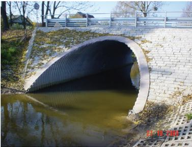
**Arch culvert.** A steel-soil multi-plate bridge/culvert on the Czarny Potok near Zamość.
