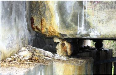
**Bearing corrosion.** A typical roller bearing works properly. However, in this case the corrosion of concrete at the end of the beam has resulted in the limit state on the extreme support.
