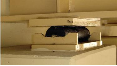
**Roller bearing.** The movable steel bearing consists of a bottom plate with a travel stopper, a roller as an articulation, a simple upper plate. The black colour of a roller comes from the graphite lubricant.
