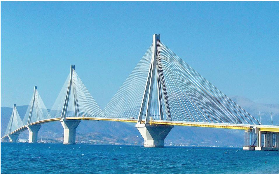
Figure 4.4.20. Rio-Antirio Bridge - combined pylon<sup>100</sup>
