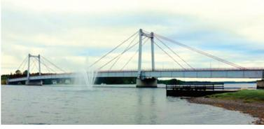
**1<sup>st</sup> cable-stayed bridge.** The Strömsund Bridge (1956) over Ströms Vattudal, constructed by Franz Dischinger. It is assumed that this is the first contemporary cable-stayed bridge.
