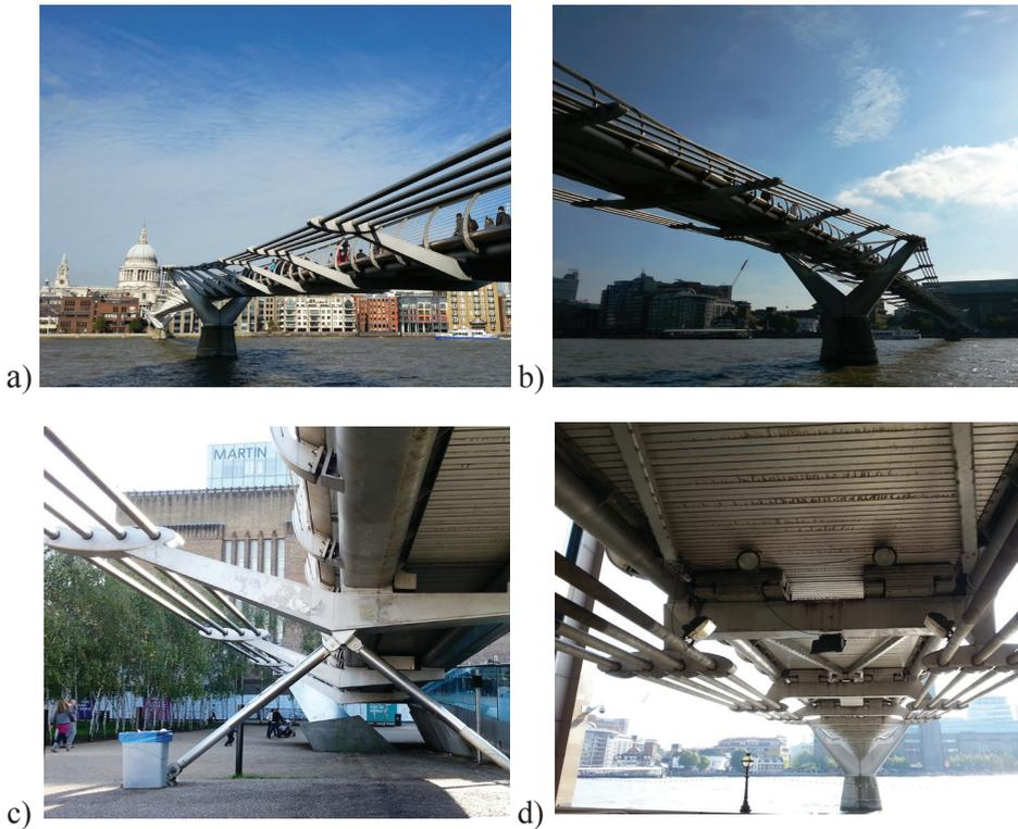
Figure 6.1. Millennium Bridge a) Suspension cables b) Deck slings to the carrying cables c) Abutment d) Mass dampers
