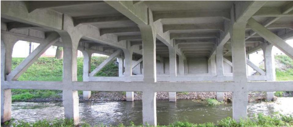
Figure 4.6.3. The bottom view on the orthotropic deck and an orderly image of pillars
