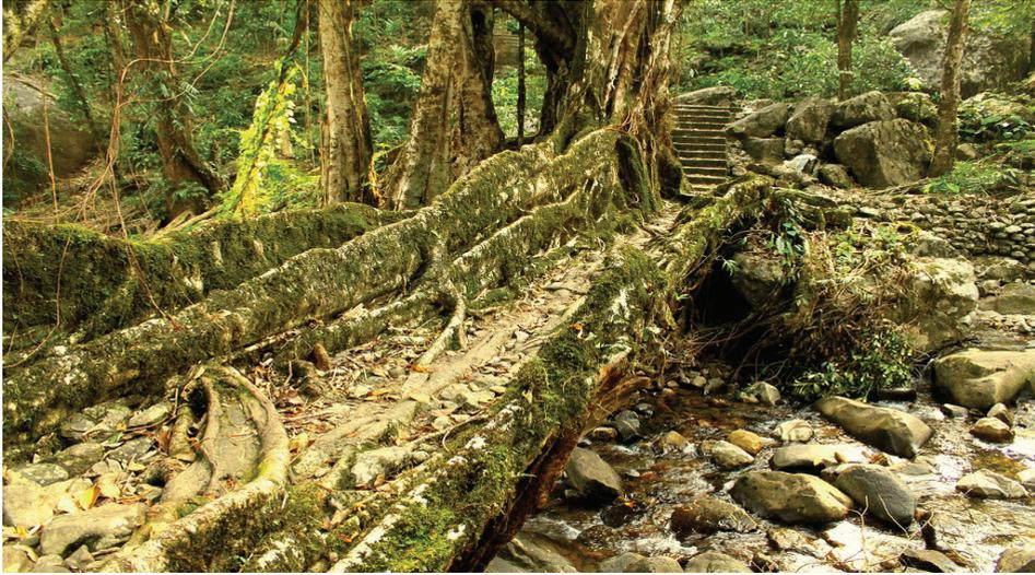
Figure 1.5.3. Surreal, strong bridge from the roots of wood; “construction” from 15 to 20 years, the older the stronger; does not require refurbishment; living bridge in Meghalya, India; source: <sup>63</sup>
