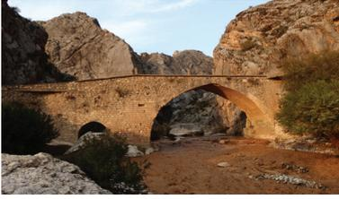
**Byzantine arch bridge.** An ancient stone bridge over the Euphrates River. A double parabolic arc is the carrying element.
