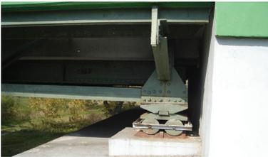
**Movable bearing.** A movable bearing of two rollers. A railway bridge.
