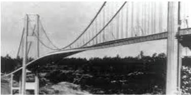
**Tacoma bridge.** Tacoma Narrows Bridge (*Galloping Gertie*) collapse in 1940. The cause of the crash was the use of significantly high plate girders of the bridge deck.
