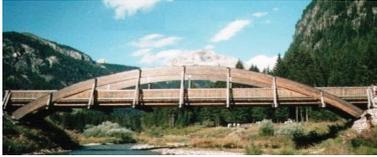
**Timber arch bridge.** A two-hinged arch bridge made of GluLam, glued and laminated timber.
