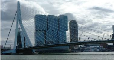
**Cable-stayed bridge.** The “deltoid” shape of pylons. Erasmusbrug (the Erasmus Bridge) over de Nieuwe Maas (1996). The west short part of the bridge works as a bascule bridge allowing the ship traffic.
