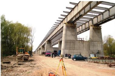
**Access wharf.** A composite superstructure under construction. The carrying element consists of two continuous tandems of steel plate-girders. The shape of the massive concrete pillars shape allows for an inspection by a trolley that moves between the columns.
