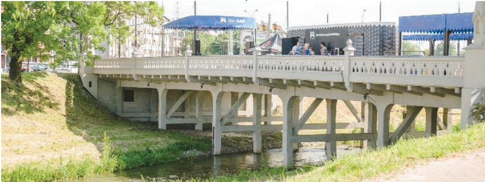
Figure 4.6.2. Lutoslawski Bridge in Lublin a) A side view b) Piles, columns and angle struts of intermediate pillars (by Monika Chmielewska)
