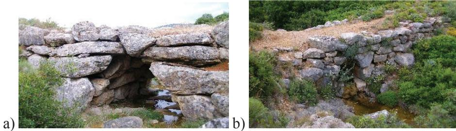
Figure 4.7.2. The Mycenaean Bridge B made with a marble blocks a) inlet b) outlet (by SLK)
