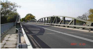
**Multi span bridge.** A bridge of the number of spans greater than 1. On the photo the outer girders have the form of arched frames..
