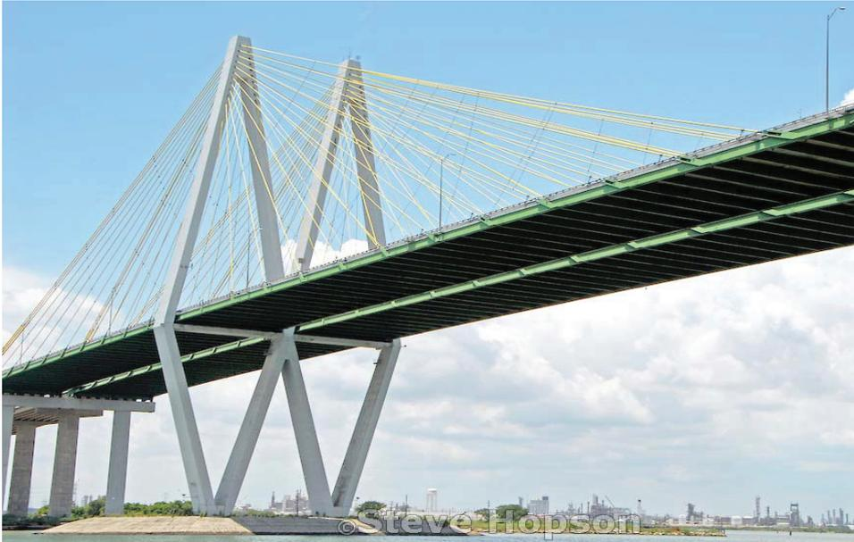
Figure 4.4.21. Fred Hartman Bridge – multiple pylon <sup>101</sup>
