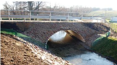
**Culvert.** Culvert – a short tunnel carrying a stream or open drain under a road or railway
