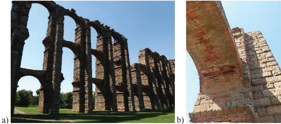
Figure 4.7.4. The Acueducto de los Milagros, 1<sup>st</sup> c. AD a) Semi-longitudinal view b) Brick arch stiffener clamped to the column of one buttress (by SLK)
