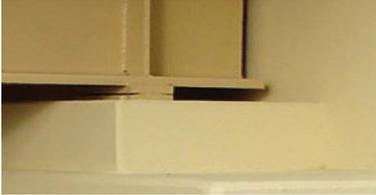
**Fixed articulated bearing.** The fixed bearing consists of a bottom plate in the form of a steel strip with a 1 cm high hummock and an upper plate. Steel bearings are simple, inexpensive and very reliable.
