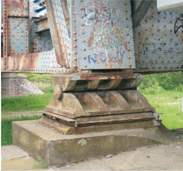
Figure 4.4.23. Articulating mounting in the foundation (*by MJ*)
