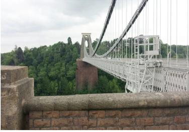
**Chain suspension bridge.** The Clifton Suspension Bridge (1864). Initially, instead of ropes, chain links with sheets of wrought iron were used. The massive pylons are made of bricks.
