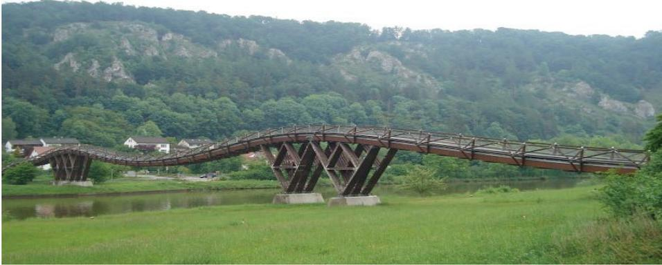
Fig. 4.8.2. Esing bridge (Essinger Brücke) – the longest wooden (GluLam) bridge (footbridge), stressed ribbon bridge in Germany (by ALT)
