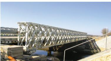
**Temporary bridge.** A temporary detour bridge, e.g. for the reconstruction period of a permanent bridge. This system was designed by Donald Bailey. It consists of prefabricated steel trusses.
