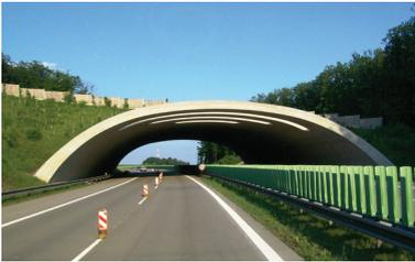
**Ecological arch bridge.** An animal upper transition on a concrete-soil arch structure, Czechia.
