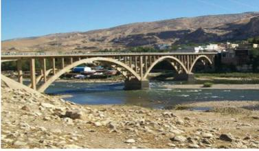
**Multi span arch bridge.** A reinforced concrete (RC) multi-span arch bridge over the Tiger River in Hasankeyf. The deck is located on arches and traffic flows on the top.
