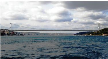
**1<sup>st</sup> Bosphorus Bridge.** Bosphorus bridge has the central span of the length at 1,074 m. The so-called low profile deck implies aerodynamic properties. Hanging cables are not vertical but stiffer zig-zag ones.
