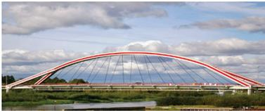
**Arch bridge.** A steel tied-arch bridge, Nielsen hangers. The bridge is of the *Barqueta* type. The bridge in Ostrołęka over the Narew River.
