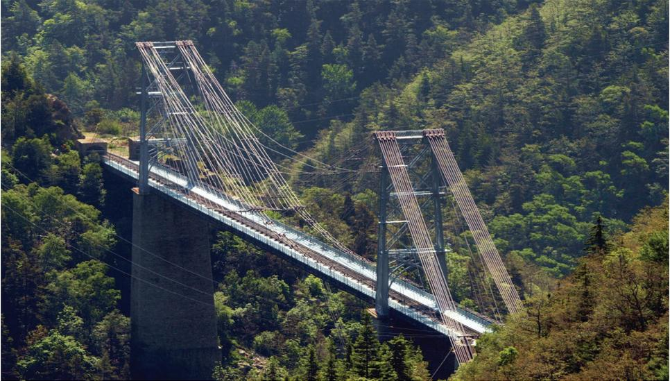
Figure 1.2.7. Pont Gisclar over the Tet river in France – railway suspension bridge; source<sup>33</sup>
