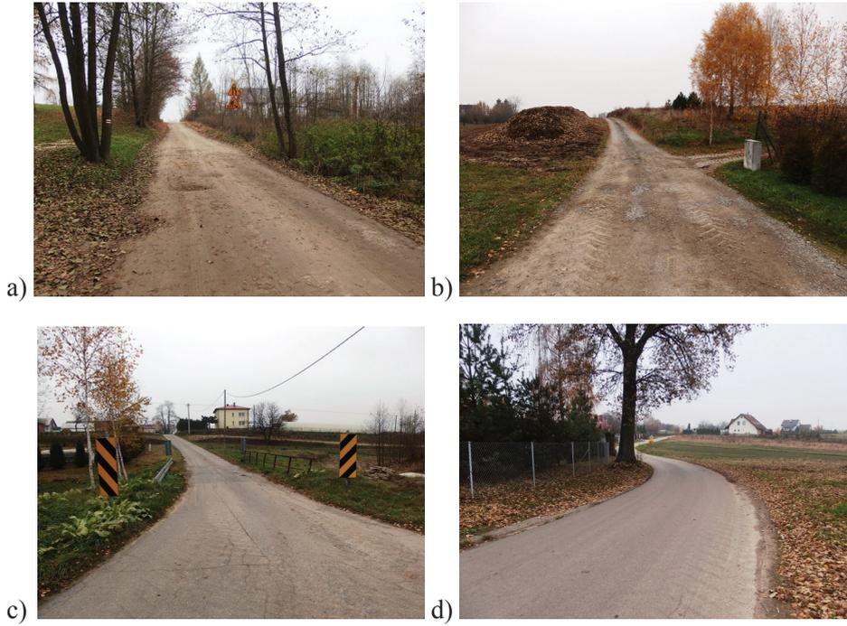
Figure 3.7.3. Rural roads a–b) gravel pavement c–d) bituminous surface, (by SLK)
