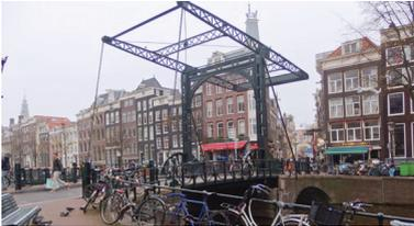
**One leaf bascule bridge.** The Staalstraat Bridge in Amsterdam, completed in 1896. A one leaf bascule bridge.
