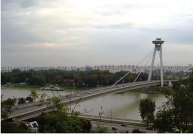
**Central cables.** The Bridge of the Slovak National Uprising (1972) over the Danube – a steel pylon and a deck where cables are fixed in the middle of the deck. A cross-section reveals a two-compartment box. Outer sidewalks on the bottom cantilevers.
