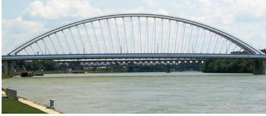
**Arch bridge.** A tied-arch bridge with radial hangers (also inclined), the Apollo bridge in Bratislava over the Danube River.
