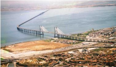
**Overpass.** The approach to the main span of Vasco da Gama Bridge (1998) in Lisbon by the multispan overpass / wharf of the length of ca. 17 km.
