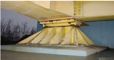
**Fixed articulated bearing.** A fixed and articulated bearing of a 50 m long railway truss bridge.
