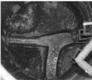
Fig. 6d. Condition: satisfactory
