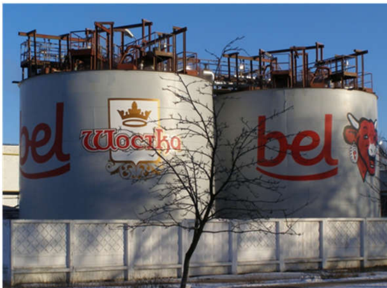
Fig. 3. Wastewater treatment plant of dairy processing plant in Shostka, Ukraine
